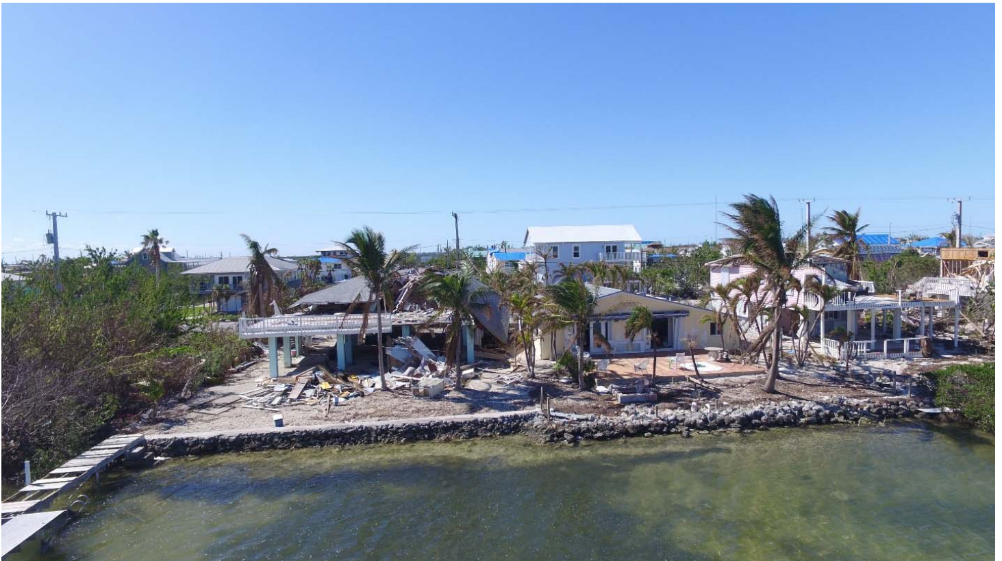
Destroyed Wood Frame Homes on Either Side of a masonry home along W Indies Drive on Ramrod Key
