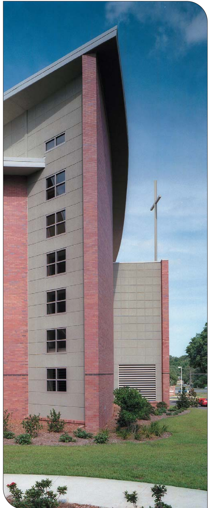
Fig. 6. A colored mortar made with light red masonry cement picks up the earth tones of this brick, while a standard gray mortar, also made with masonry cement, complements the concrete masonry units that it joins. (IMG14575)
