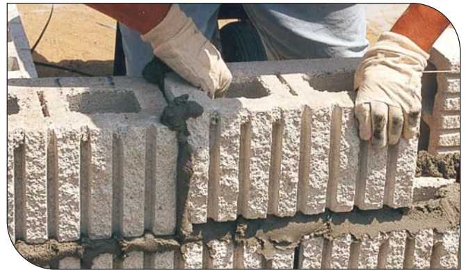
Fig. 1. Mortar of proper workability is soft, but with good body; it spreads readily and extrudes without smearing or dropping away. (IMG13629)
