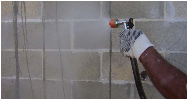
Figure 3 - Uniformly wetting the wall
