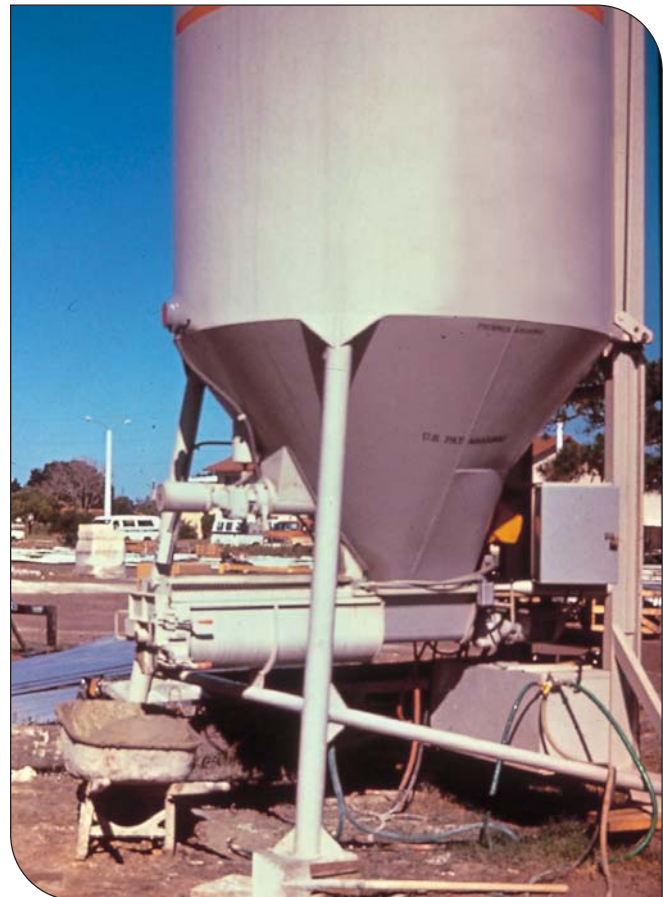
Fig. 14. When connected to electricity and water at the jobsite, the silo mixer is ready to produce mortar as needed. (IMG14096)
