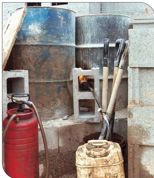
Figs. 11a, b. Warm sand and a continuous supply of hot water may be needed when cold weather arrives. Sand can be heated over fire in a pipe (above) and water can be heated in metal drums (below). (IMG12506, IMG12507)
