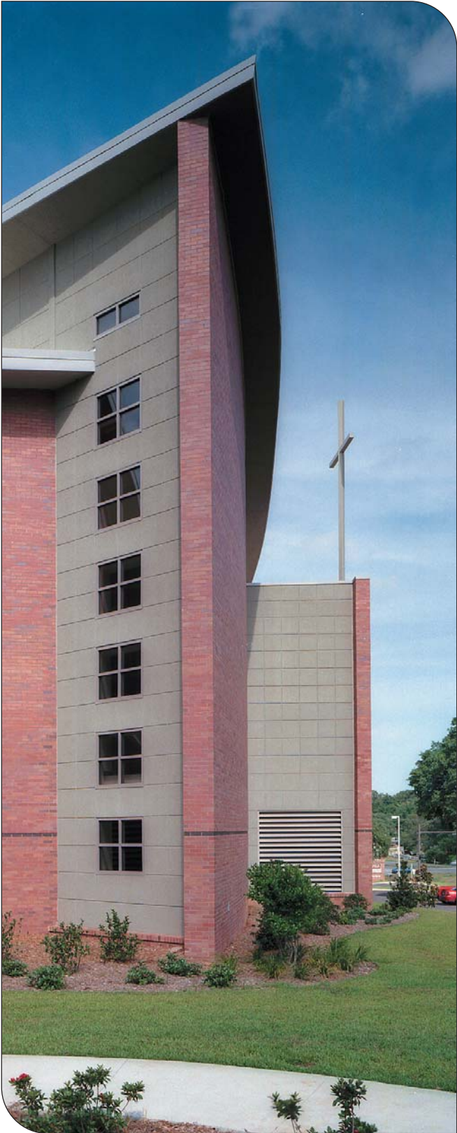
Fig. 6. A colored mortar made with light red masonry cement picks up the earth tones of this brick, while a standard gray mortar, also made with masonry cement, complements the concrete masonry units that it joins. (IMG14575)
