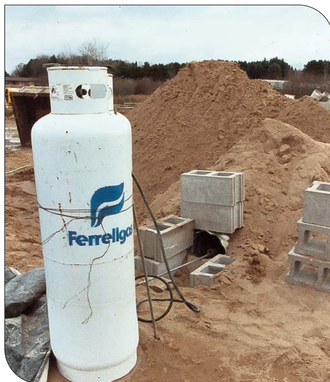
Figs. 11a, b. Warm sand and a continuous supply of hot water may be needed when cold weather arrives. Sand can be heated over fire in a pipe (above) and water can be heated in metal drums (below). (IMG12506, IMG12507)
