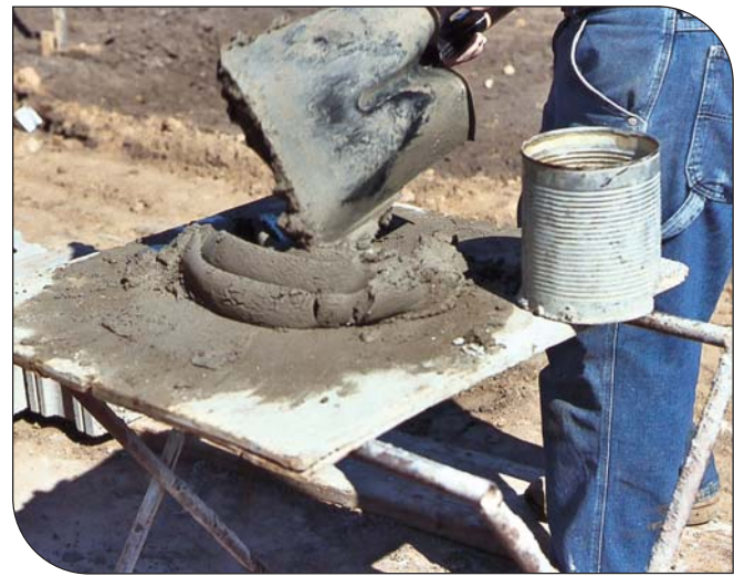
Fig. 10. To restore workability, mortar may be retempered. (IMG13630)
