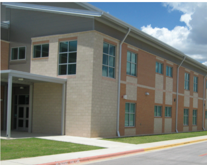
Masonry school #20 east side view
