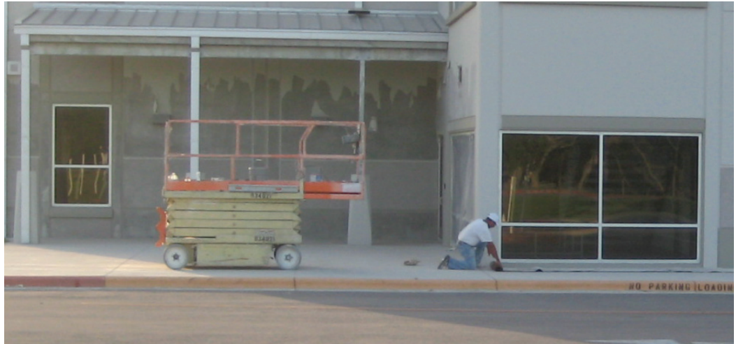
Tilt-up school #22 repainting
