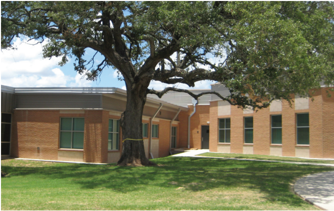
Masonry school #20 west side view
