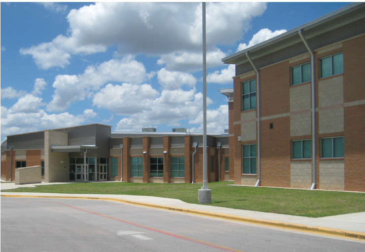
Masonry school #20 front view
