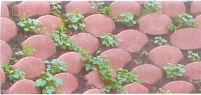
Concrete hardscape products filter stormwater run-off and support grass or other plant growth with open cell product designs.
